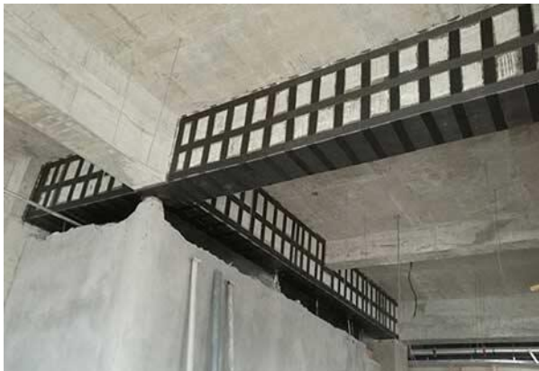
Figure 1 FRP Wrapped Beam
