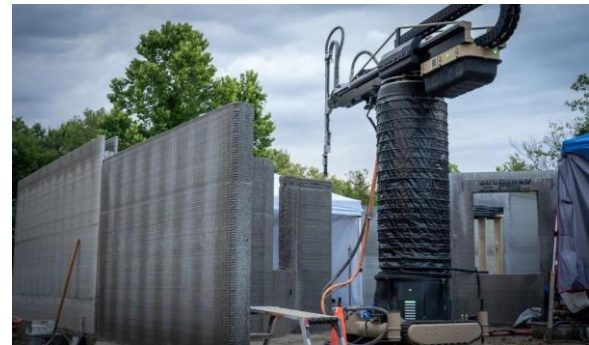
Figure 2 Typical Printed Wall
